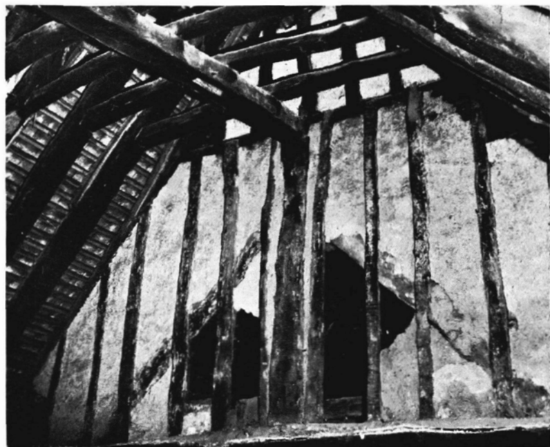
B. Upper part of North-west side of Partition between Hall and Room above Service.
