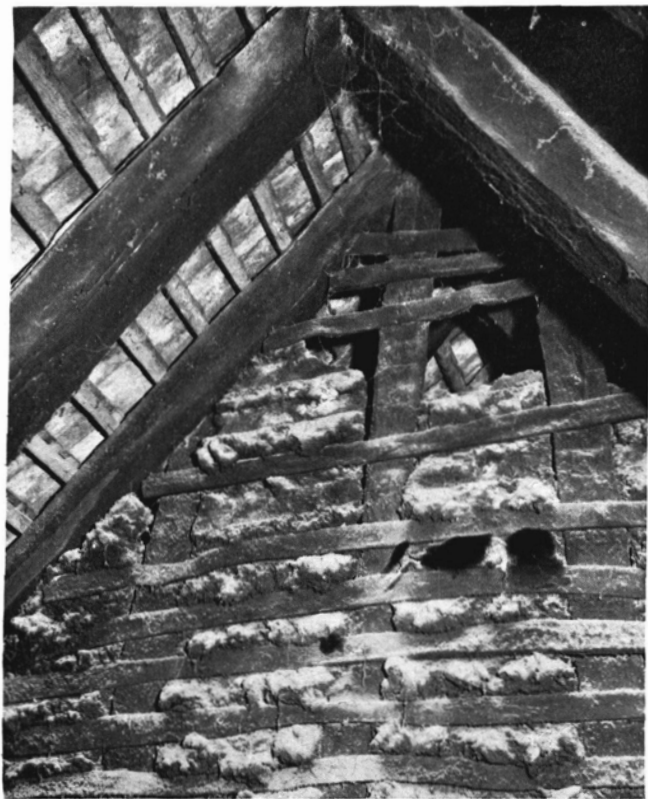
A. Space above Collar on line of Service Truss, showing Daub Filling unsmoothed towards Hall.
